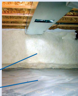
Insulated crawl space wall
