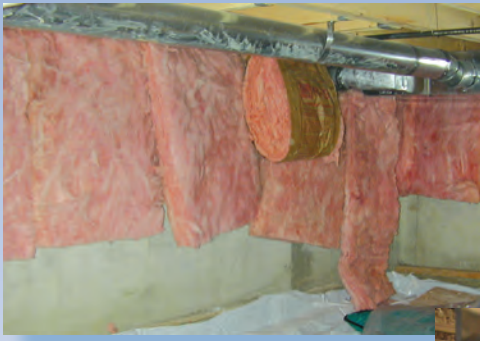
As the result of outdated understanding and insufficient attention to details, many crawl spaces built in the past have not performed well. The left photo shows insulation installation practices that were haphazard at best. New approaches treat crawl spaces as conditioned spaces, with quality insulation work, moisture control and heat delivery (right).
