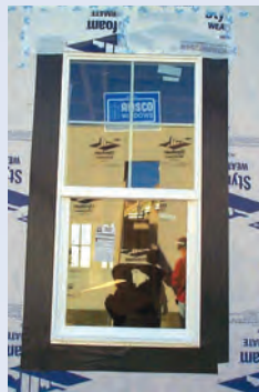
Drainage plane materials include exterior foam sheathing with taped joints (left), building paper and flashing around windows and doors (right). Neither typical wood-based sheathings nor exposed caulk are appropriate choices. Installation details are critical.
