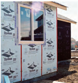
Drainage plane materials include exterior foam sheathing with taped joints (left), building paper and flashing around windows and doors (right). Neither typical wood-based sheathings nor exposed caulk are appropriate choices. Installation details are critical.
